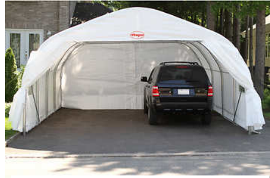
Figure 3.19: Temporary Car Shelter
